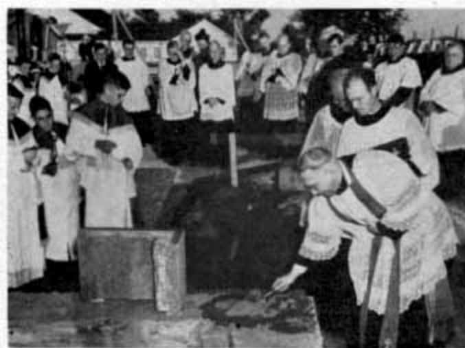
CORNERSTONE IS LAID
